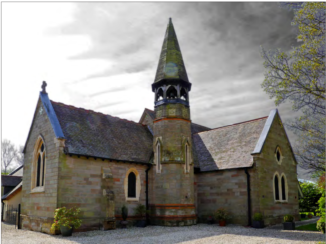
Former Blackwell church – now a live-work unit
